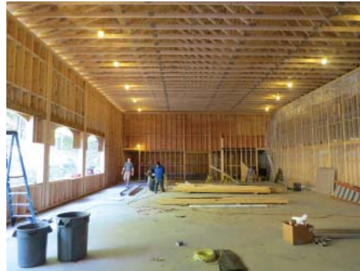
Interior framing almost done
