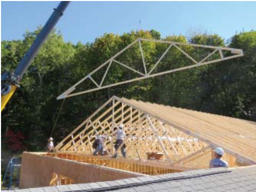
Trusses being installed
