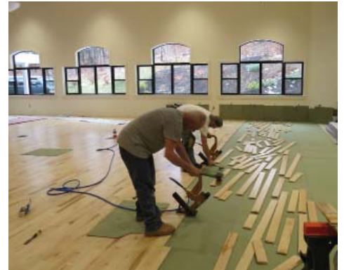
The final step ~ installing the floor
