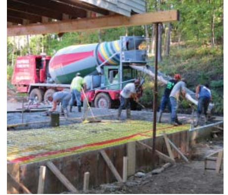
Laying the cement slab
